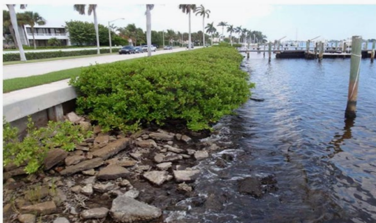
Figure A.6: Example of 7ft Sea Wall with Living Shoreline
